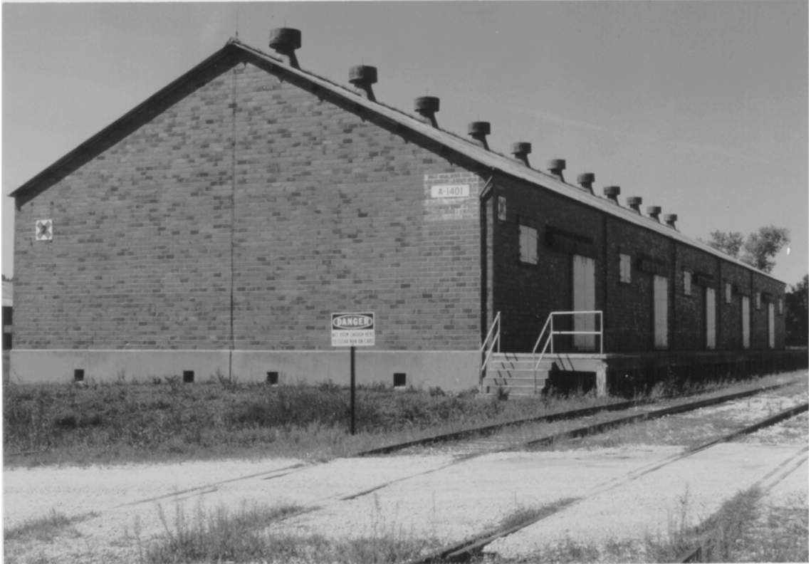
Figure 27. Hollow clay tile aboveground magazine.
