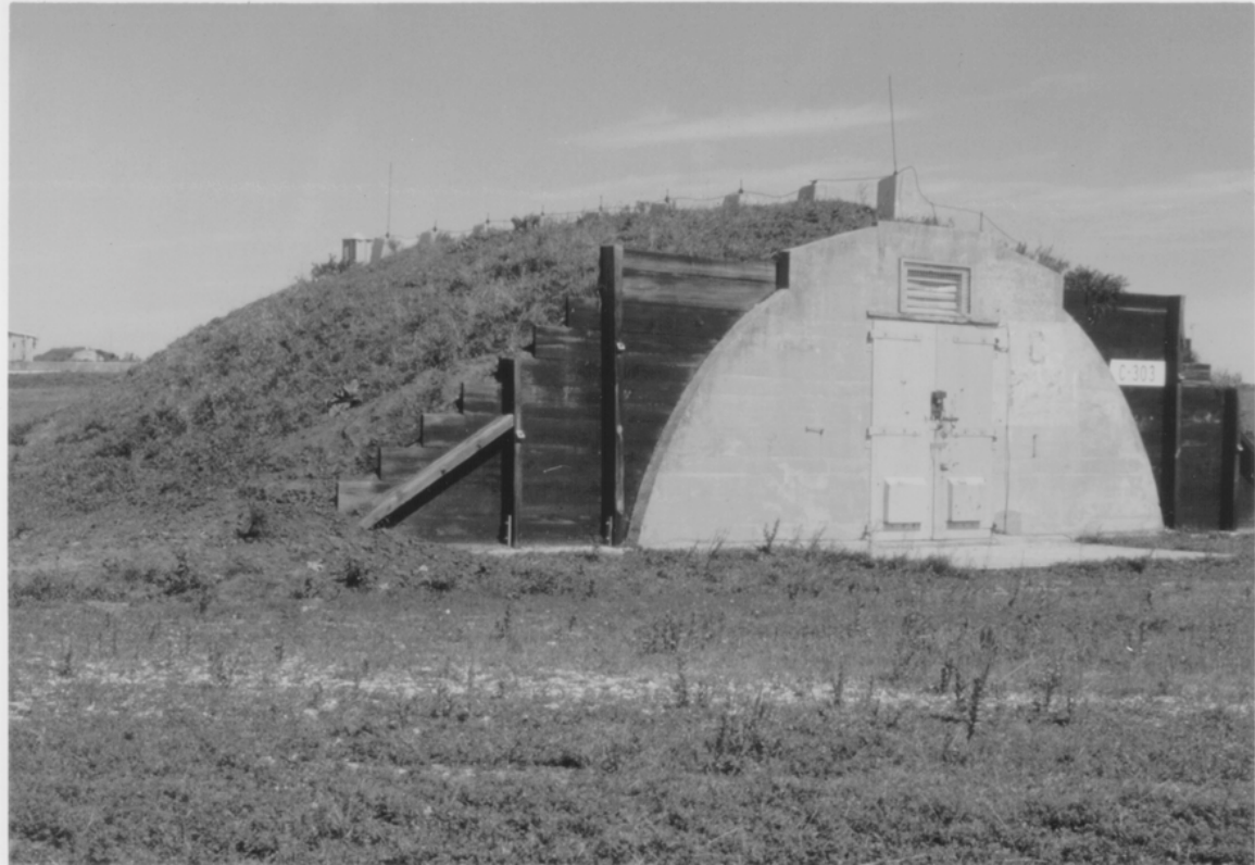
Figure 14. Standard underground magazine at Savanna Army Depot.
