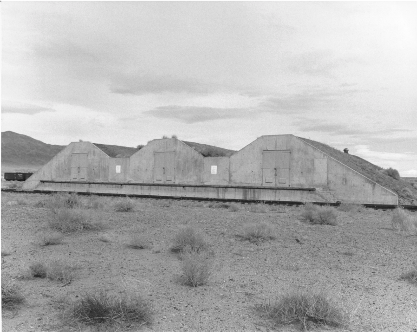
Figure 11. Triple Arch Magazine at Hawthorne Naval Ammunition Depot.
