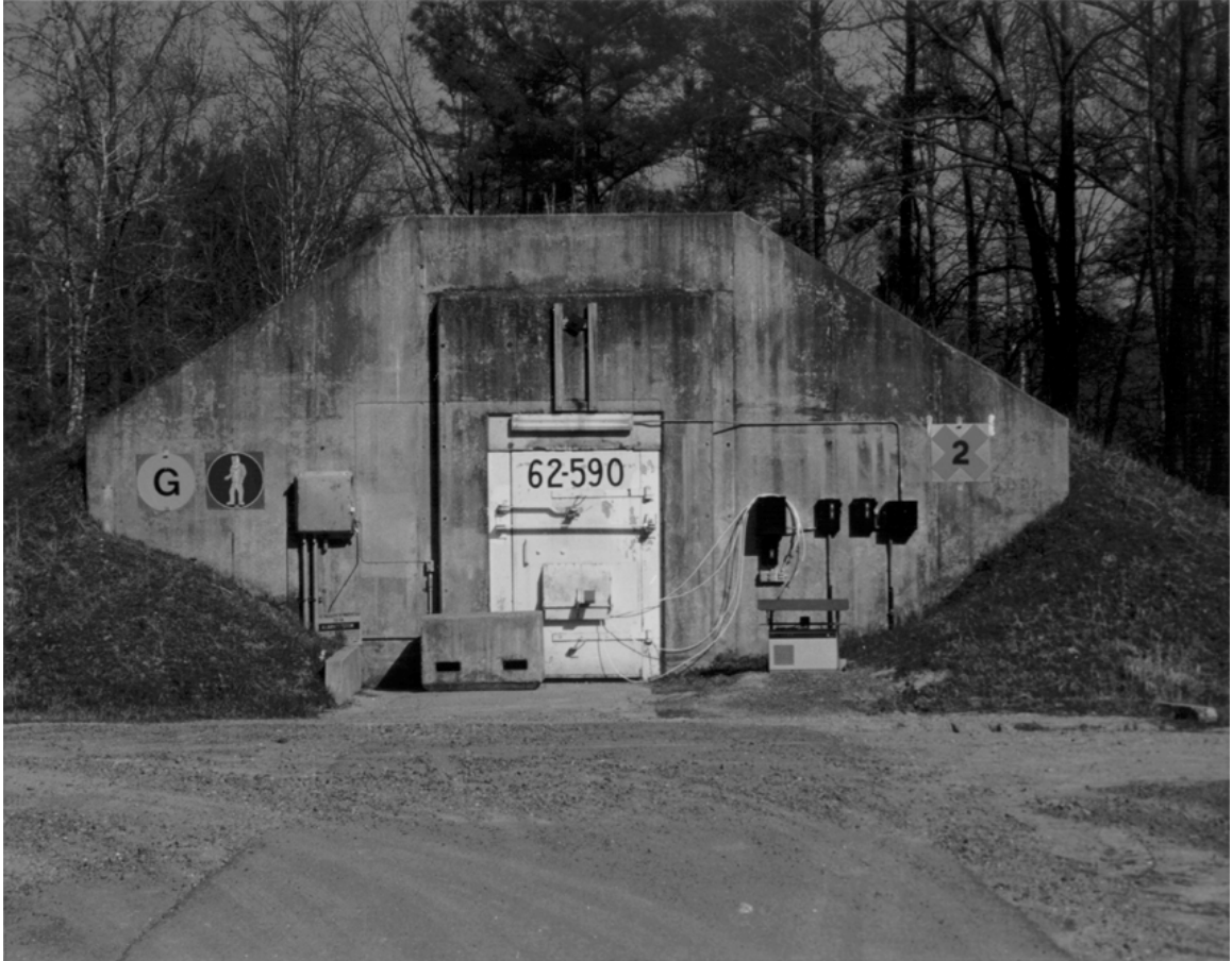
Figure 24. Igloo at Pine Bluff Arsenal that has been modified with refrigeration for biological weapons storage.
