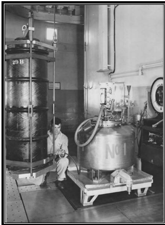
Plate 5.20 Nitroglycerin dessicator with technician connecting ground wire (Photo courtesy US Army)
