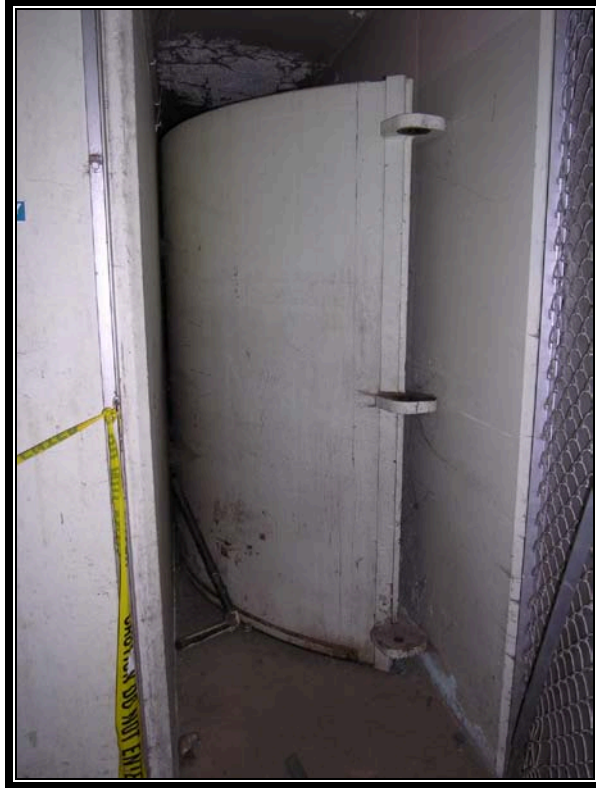
Plate 5.67 Original door stored in personnel passage (Photo courtesy US Army, 2007)
