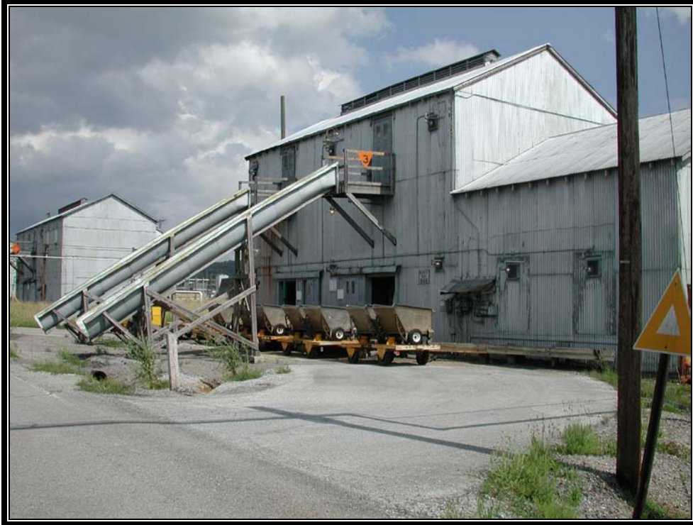
Plate 5.7 Typical air dry building (Photo courtesy US Army)
