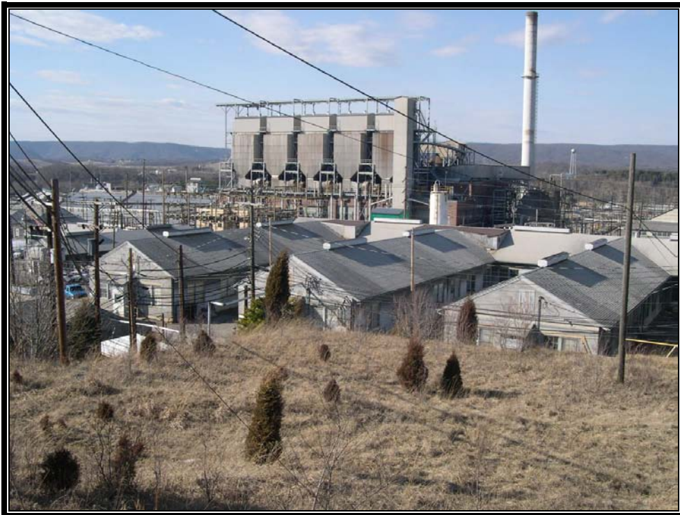
Plate 5.36 Example of a steam generating plant with World War II administration building (now demolished) in foreground (Photo courtesy US Army)
