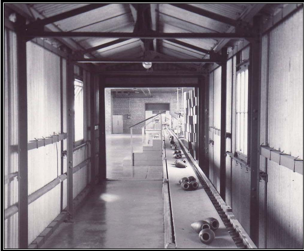
Plate 5.54 Typical ramp with conveyor, ca. 1943 (Photo courtesy US Army)
