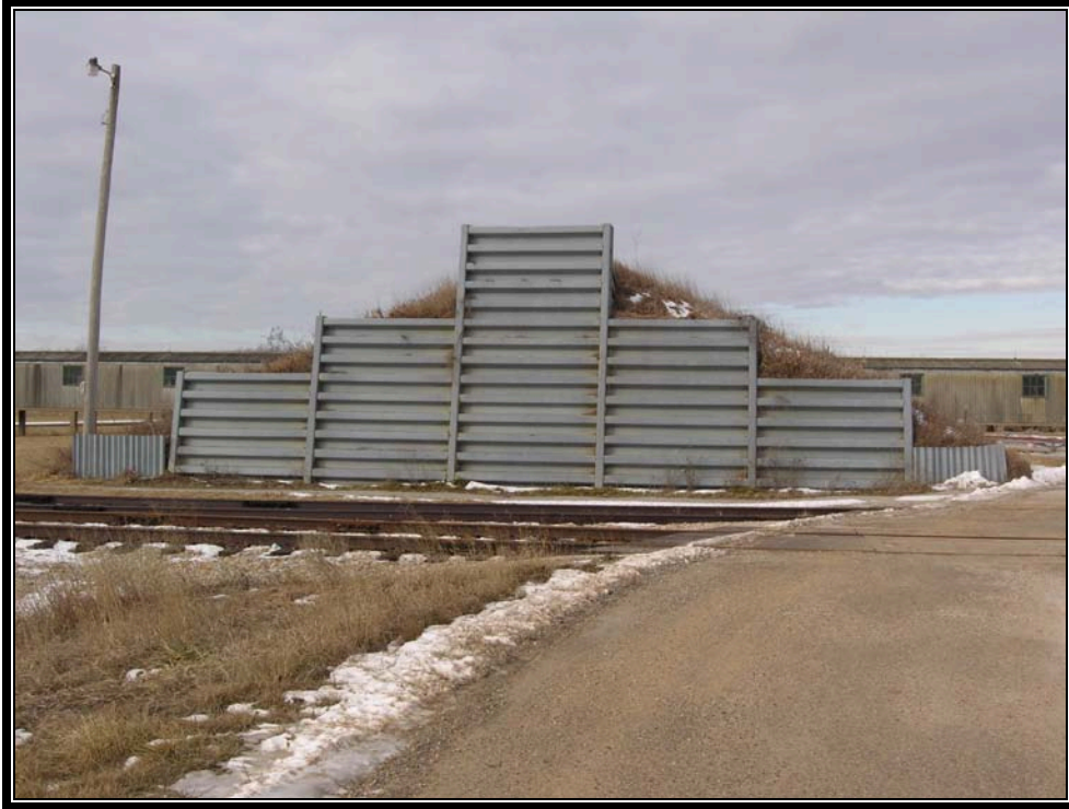
Plate 5.43 Typical barricade (Photo courtesy US Army, 2007)
