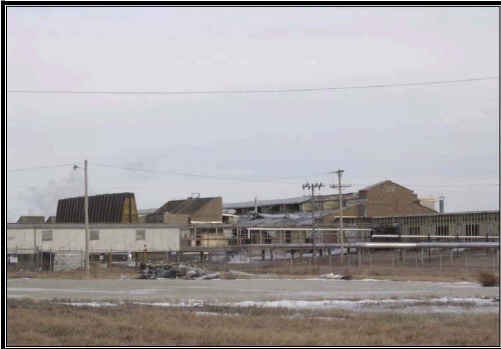
Plate 5.66 Renovated building. Note large concrete machining bays and barricade near center of building (Photo courtesy US Army, 2007)
