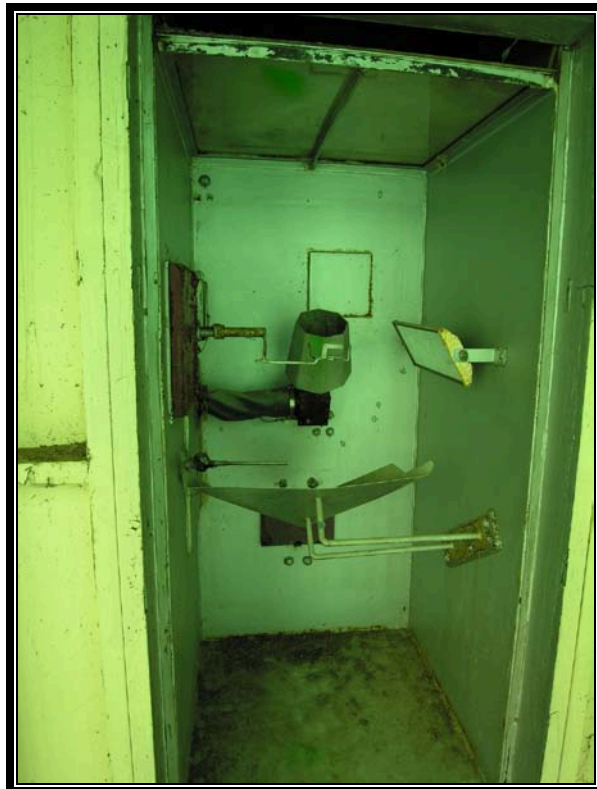
Plate 5.50 Typical concrete cell for remote testing of detonators (Photo courtesy US Army, 2007)
