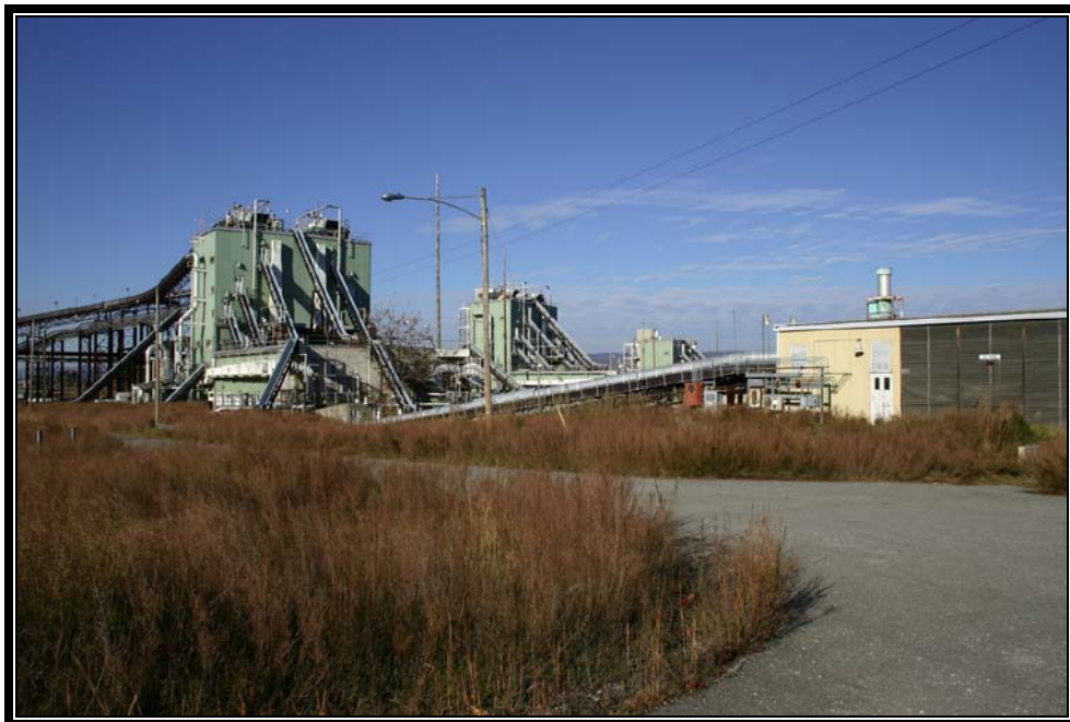
Plate 5.30 Typical Continuous Automated Multi-Base Propellant Line (CAMBL) (Photo courtesy US Army)
