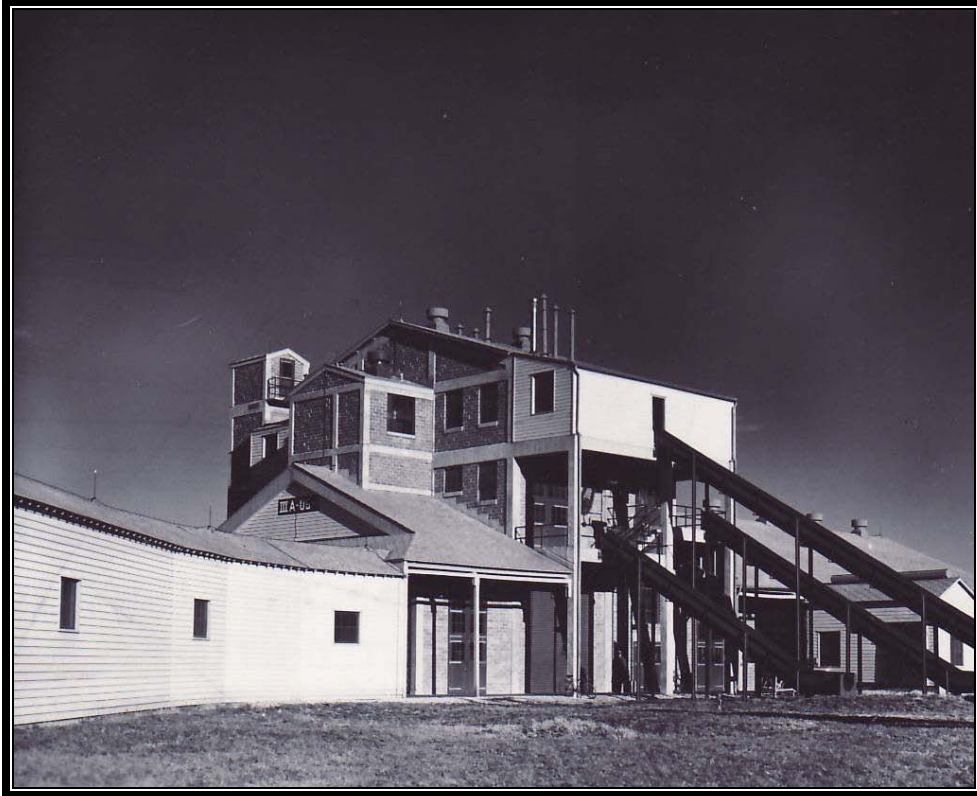
Plate 5.41 Typical melt pour building, ca. 1943 (Photo courtesy US Army)
