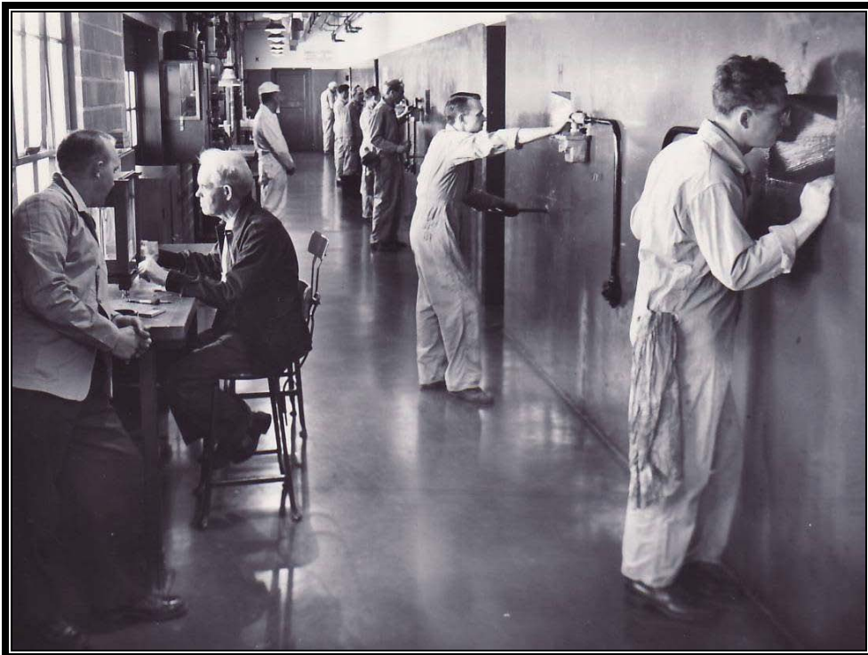
Plate 5.48 Typical concrete barricade for remote assembly of boosters, ca. 1943, (Photo courtesy US Army)
