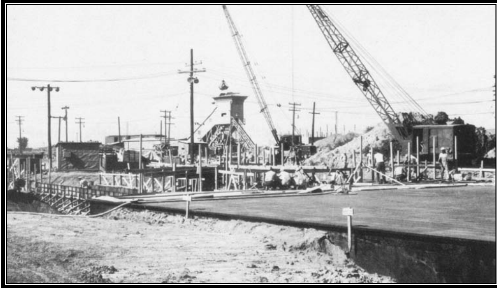
Plate 5.63 Construction of underground complex of buildings, ca. 1951 (Photo courtesy US Army)
