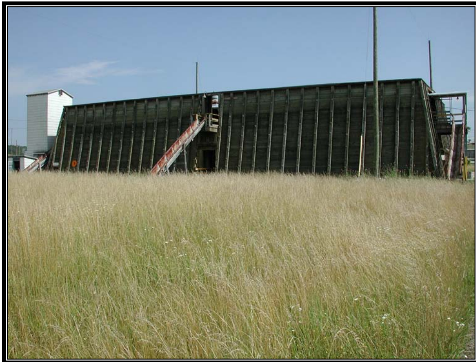
Plate 5.6 Typical solvent recovery building surrounded by Rapauno barricade (Photo courtesy US Army)
