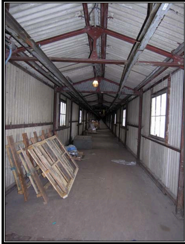
Plate 5.55 Typical ramp with conveyor removed (Photo courtesy US Army, 2007)
