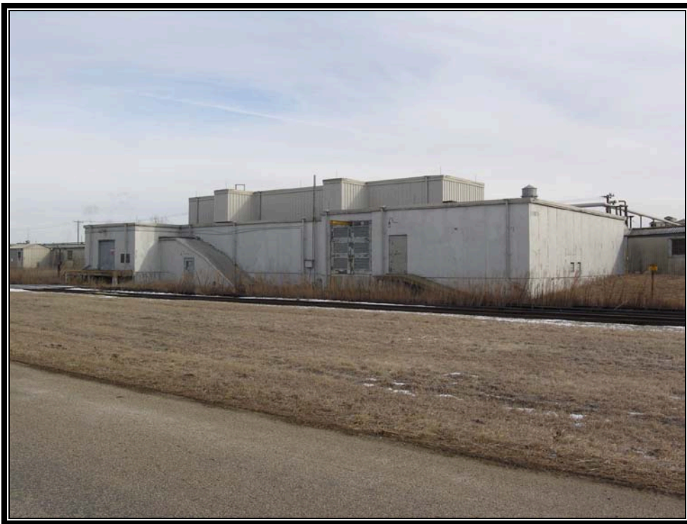
Plate 5.64 Example of explosives handling facility (Photo courtesy US Army, 2007)
