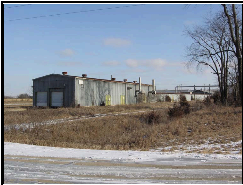
Plate 5.70 Example of utilitarian nature of later construction (ca. 1968) emphasizing economy rather than architectural style (Photo courtesy US Army, 2007)
