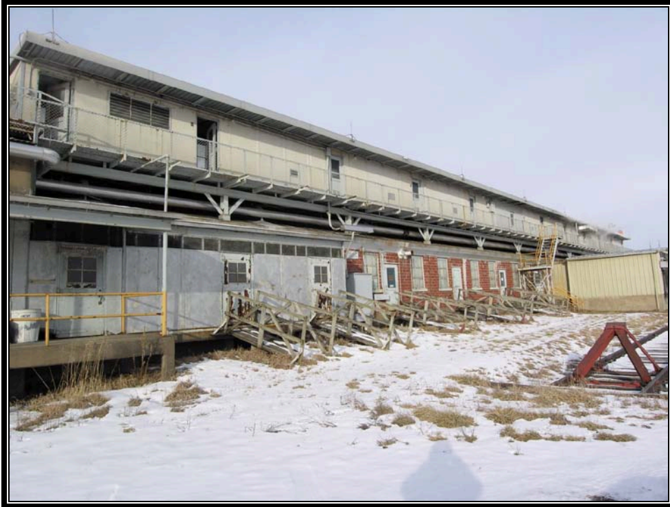
Plate 5.65 Typical method of installing air conditioning ductwork (Photo courtesy US Army, 2007)
