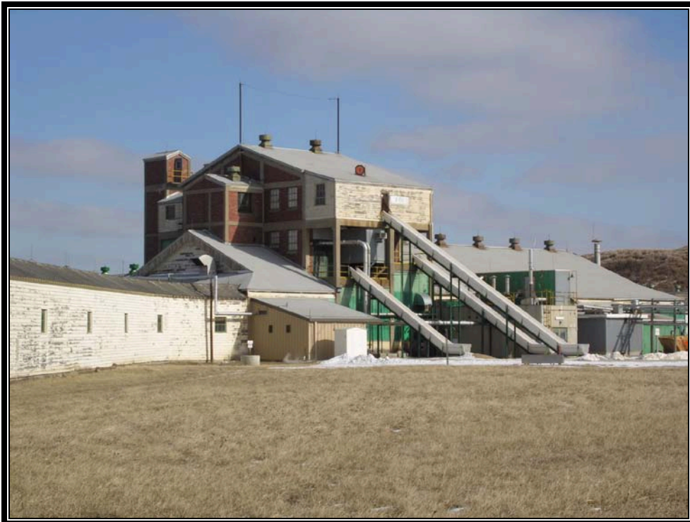
Plate 5.44 Typical melt-pour building (Photo courtesy US Army, 2007)
