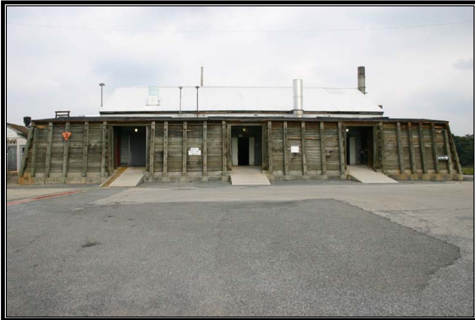
Plate 5.18 Typical building where cutting and cellulose wrap are completed, note Repauno barricade (Photo courtesy US Army)
