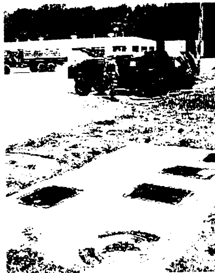
Photo 3-1. Pre-constructed OWS installed at a new motor pool washrack location. All the new OWS were equipped with small manways, inhibiting access to the internal chamber and removal of the coalescing tube packs.
