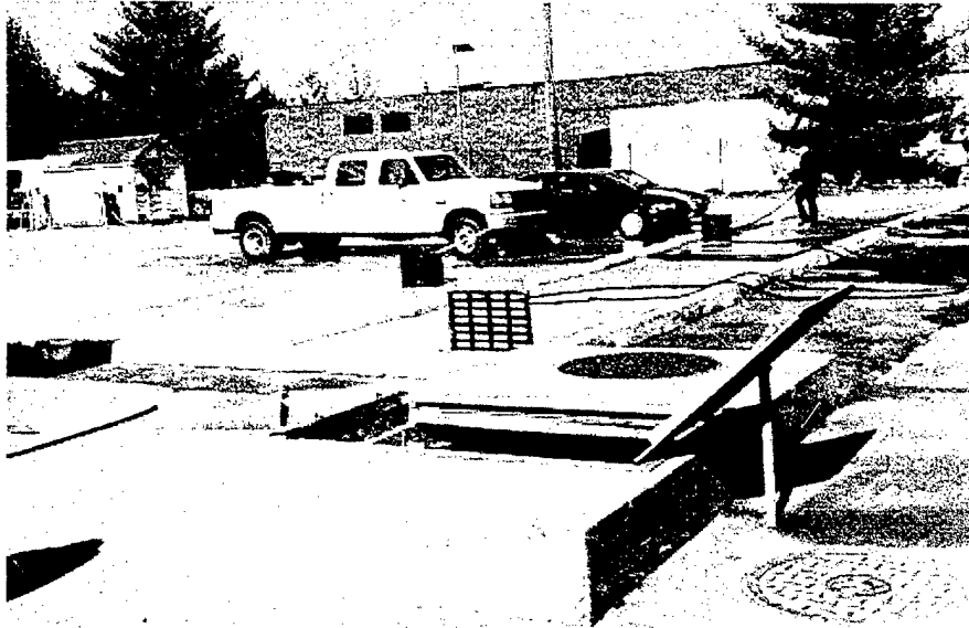
Photo 3-2. OWS at TMP site with its door panels open. All the retrofitted OWS were equipped with similar door panels, allowing easy access to the coalescing tube packs.
