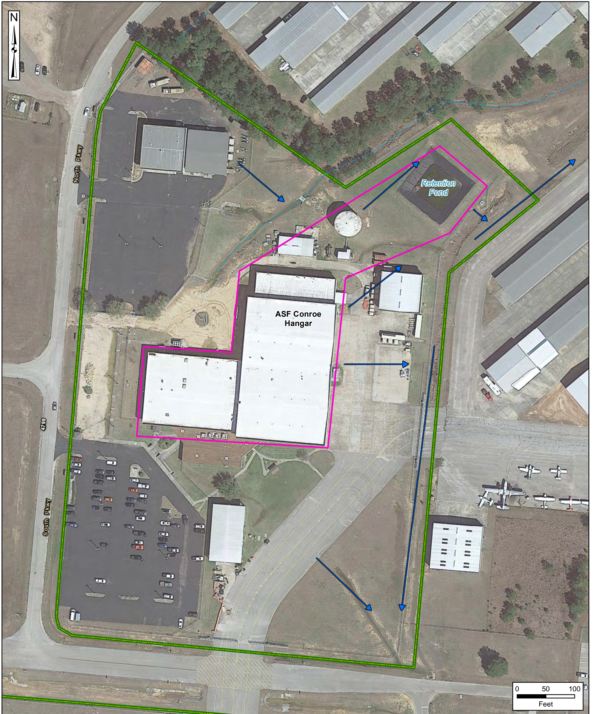
Figure 5-2 Aerial Photo of ASF Conroe Hangar
