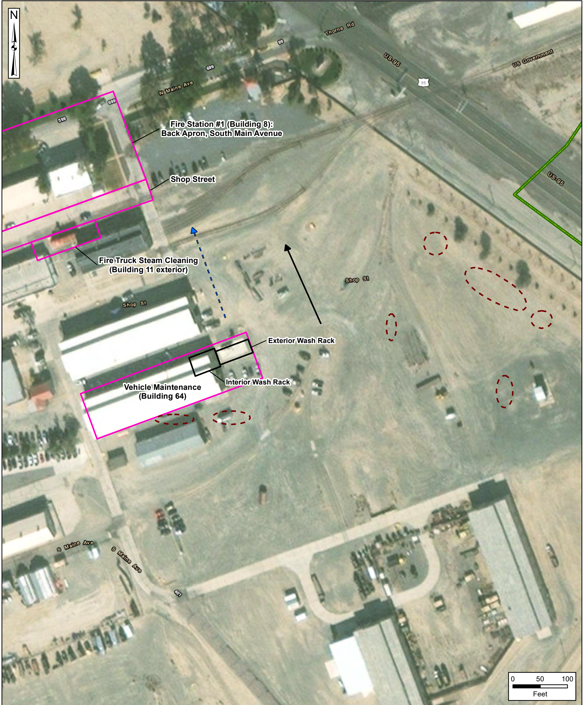
Figure 5-10 Aerial Photo of Vehicle Maintenance (Building 64)
