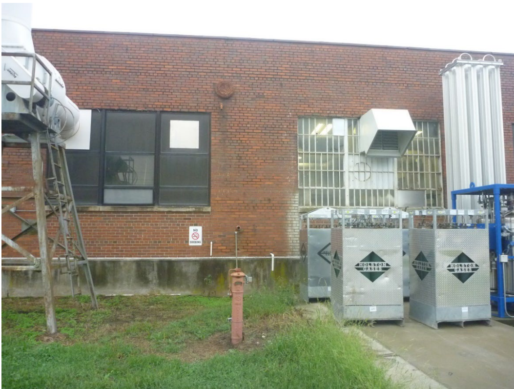
Photograph D-2. Exterior of Building H (C Bay) Facing South
