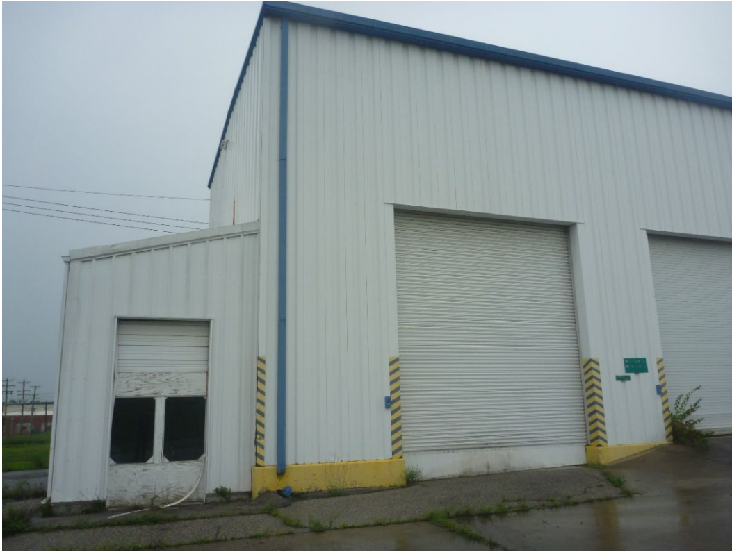
Photograph D-5. East End of Building 105 Exterior Facing South
