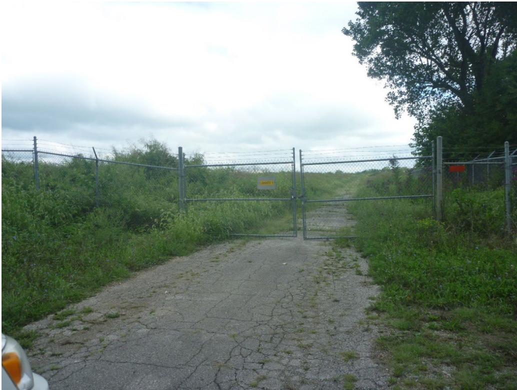
Photograph D-16. Entrance to New landfill Facing North
