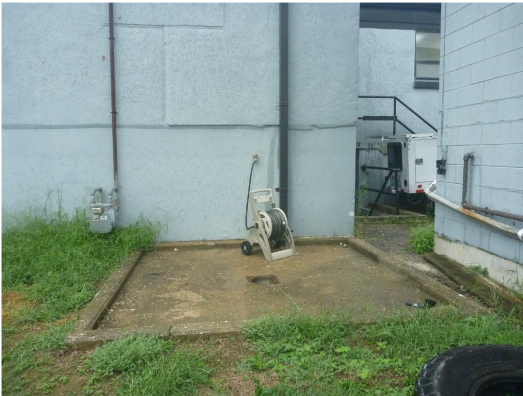
Photograph D-4. Wash Rack Area of Building 30
