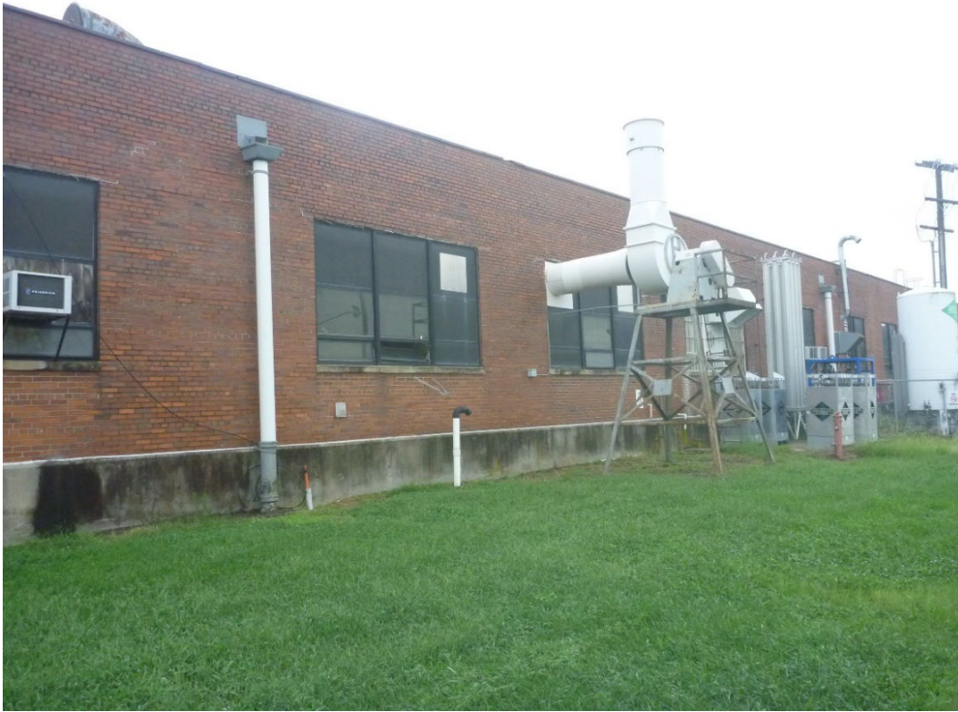
Photograph D-1. Exterior of Building H (C Bay) Facing Southwest
