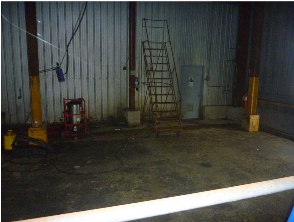
Photograph D-8. Interior of Building 105 Showing Trench Drains Facing East
