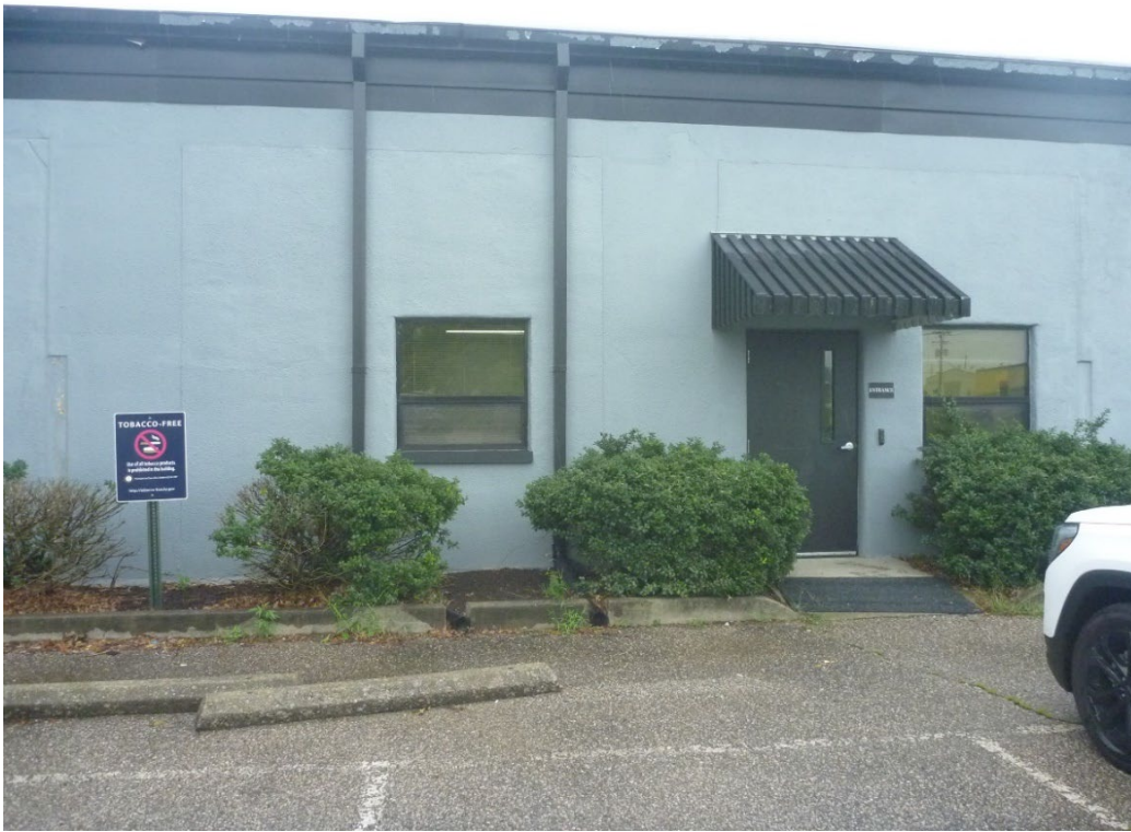
Photograph D-3. Front of Building 30 Showing Garage Bays of Former Fire Station
