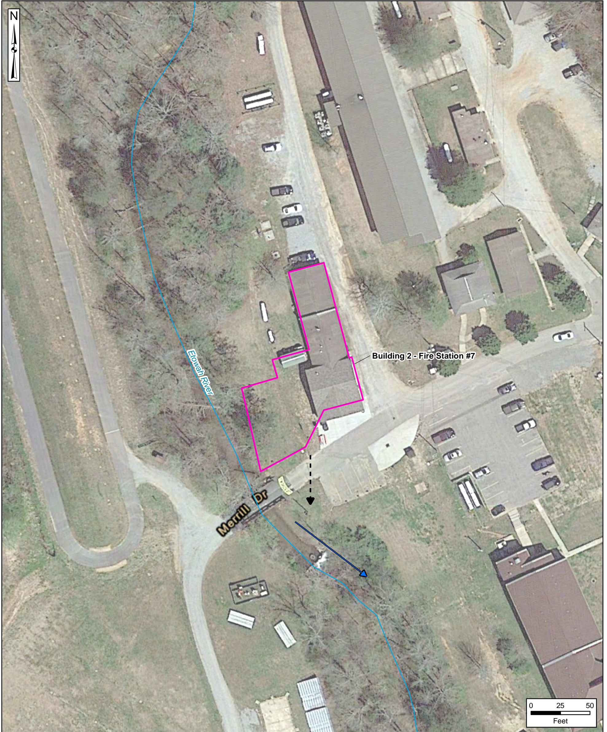
Figure 5-3 Aerial Photo of Building 2 - Fire Station #7 AOPI
