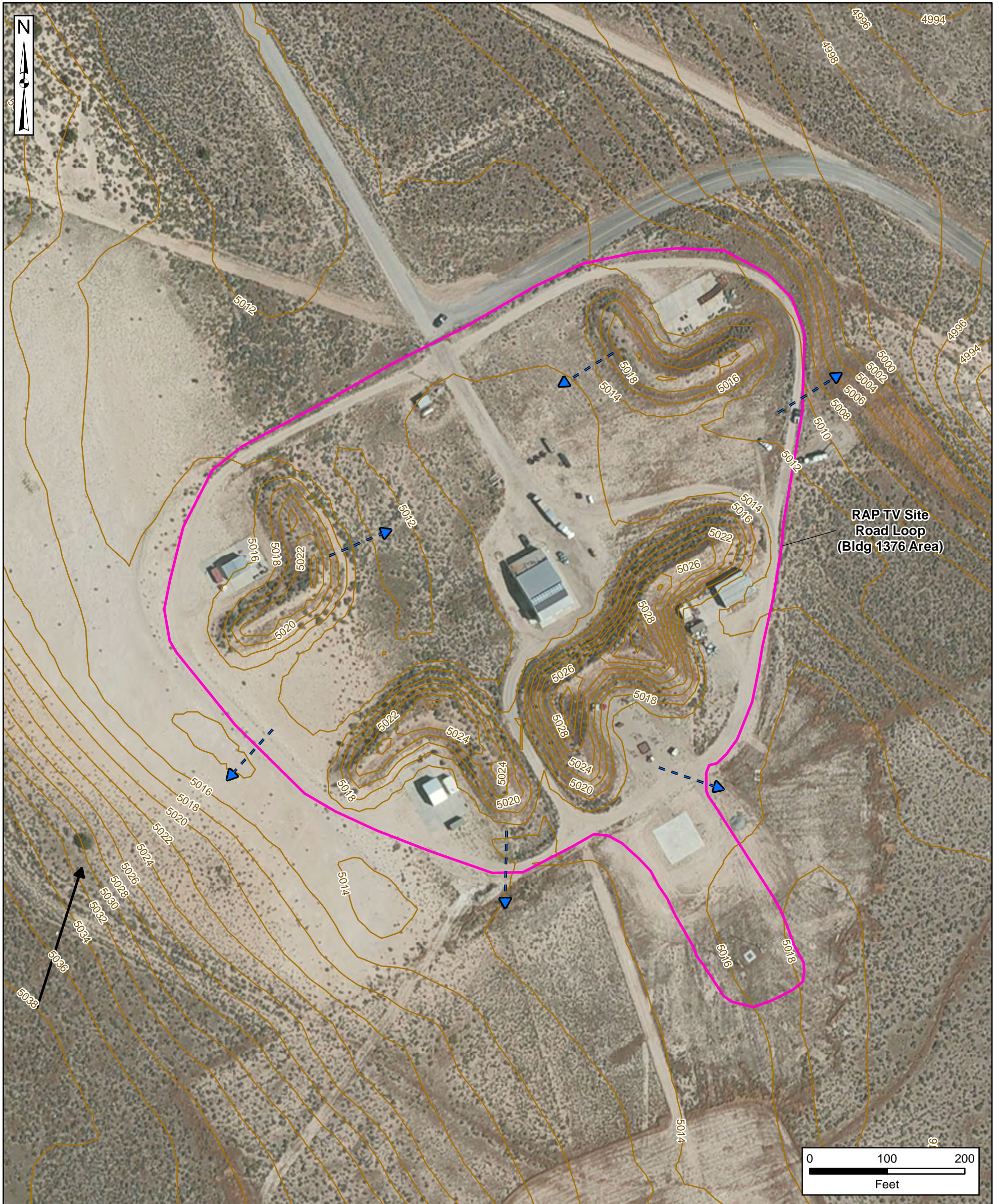
Figure 5-8 Aerial Photo of RAP TV Site Road Loop (Building 1376 Area) AOPI
