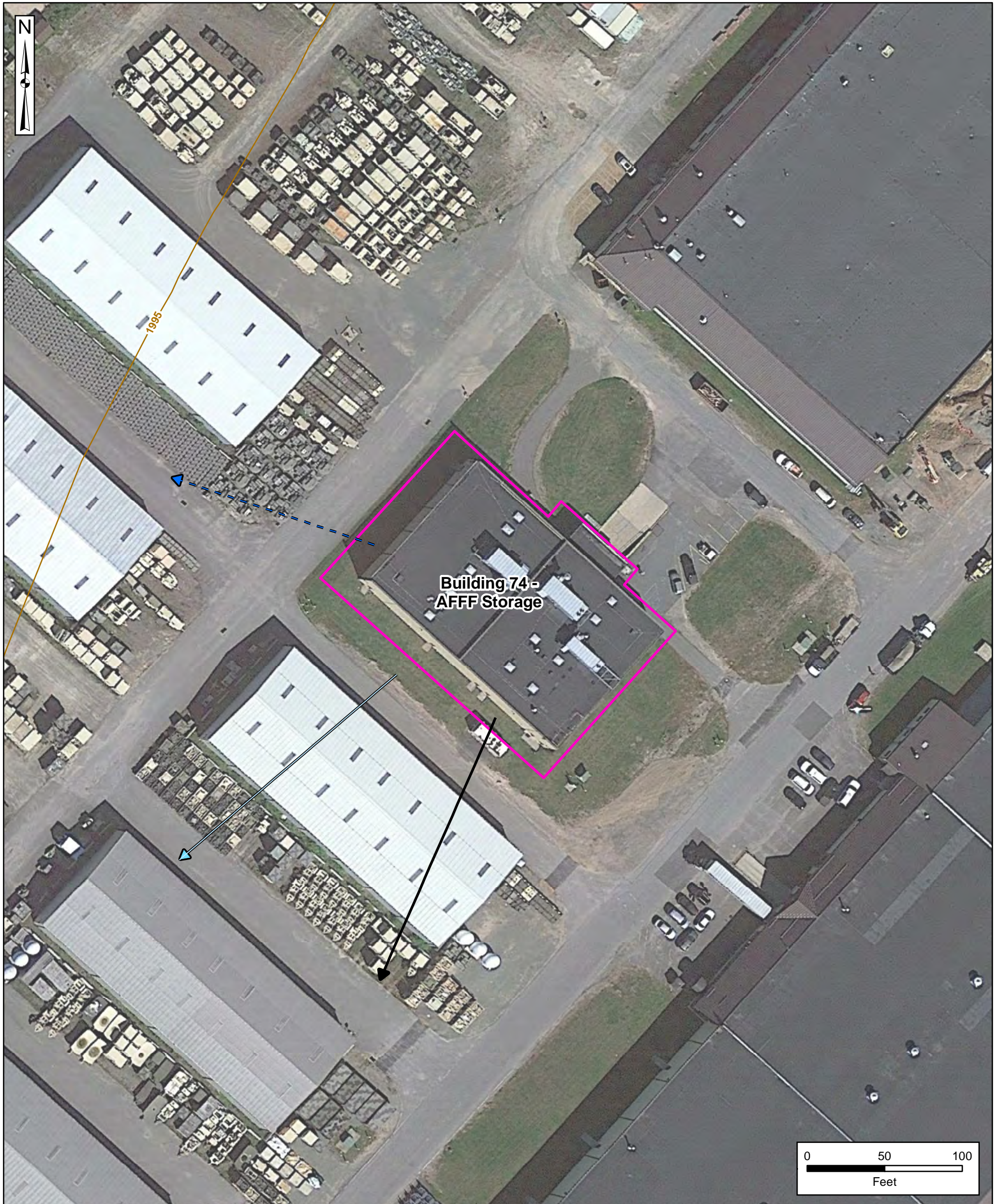
Figure 5-9 Aerial Photo of Building 74 - AFFF Storage
