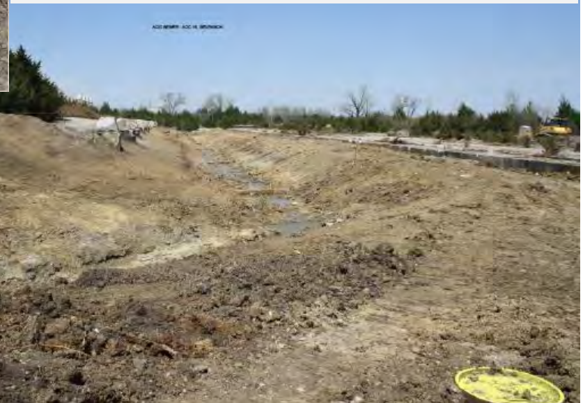
E Line Acid Sewer Removal - During
