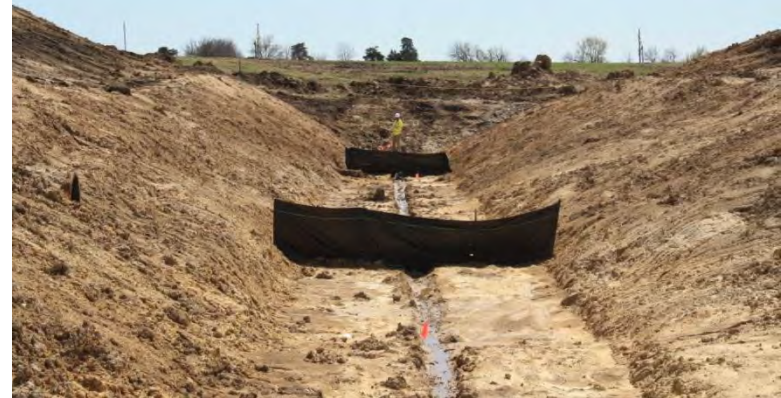
SWMU 26 - Sewer Removal
