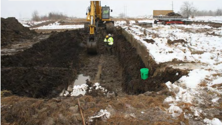
SWMU 26 - Sewer Removal
