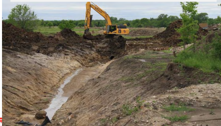
SWMU 26 – Sewer Removal
