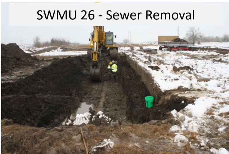
SWMU 26 – Sewer Removal
