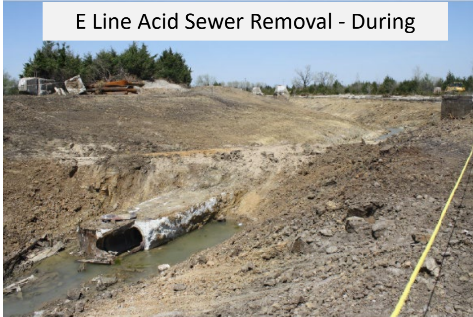
E Line Acid Sewer Removal - During
