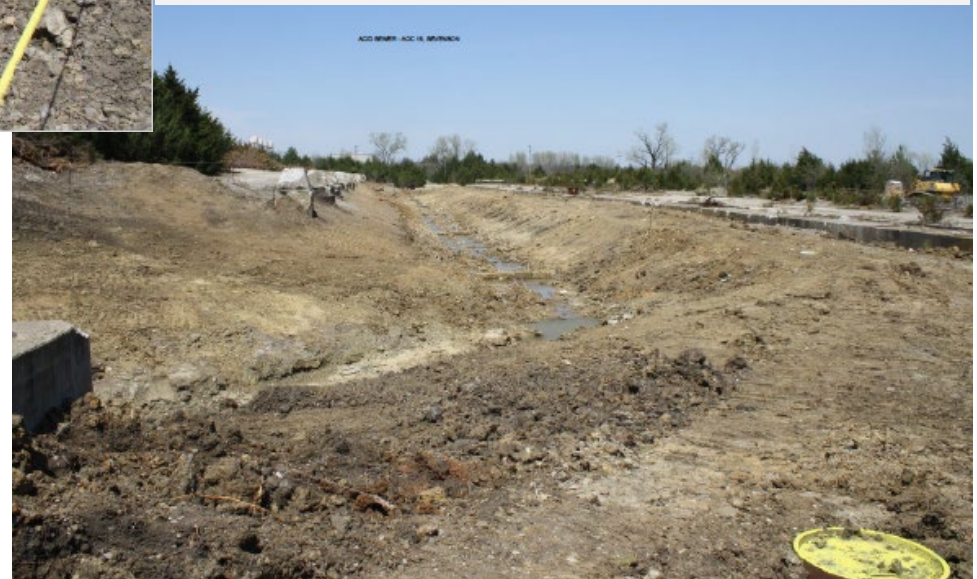
E Line Acid Sewer Removal - During
