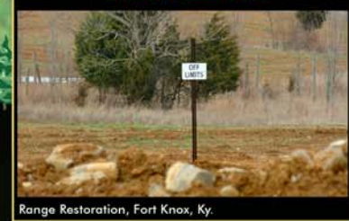
Range Restoration, Fort Knox, Ky.
