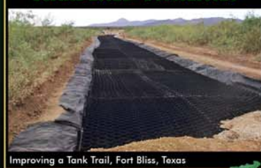
Improving a Tank Trail, Fort Bliss, Texas
